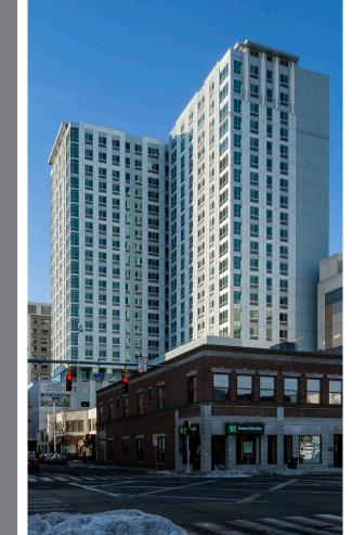
Erland constructed this mixed-use high-rise rental housing development on a complex, tight site in downtown Stamford. We began by demolishing an existing building. Steel had to be erected over the top of an adjacent, functioning restaurant.
