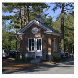
The Andover Companies Guard House and Dining Renovations scope included the construction of a new 16x16ft guard house constructed following the same program of the new Wellness Center and existing building. It utilized the same granite and brick masonry veneers, elegant exterior architectural trim, and slate roofing to match the rest of the campus.
